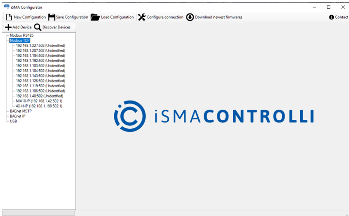
Figure 23. Devices discovered via Modbus TCP/IP
